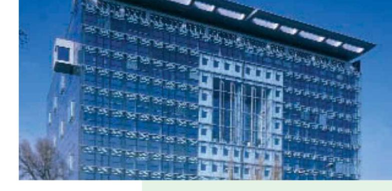
Pilkington Suncool™ High Performance is a range of off-line coated, energy management glass combining high light transmission with solar control performance. It is always used as part of an insulating glass unit – or a Pilkington Planar™ system – where its coating also provides the highest level of thermal insulation. A range of colours including clear, neutral, silver and coloured tints is available, as well as a self-cleaning version – Pilkington Activ Suncool™.
