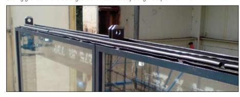
Lifting & Lining plates: Fitted to top corner of frame to allow for lifting during transport and installation.
