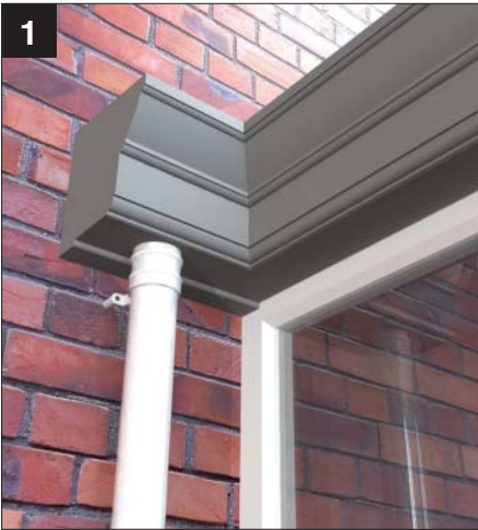
Return back to house wall applies to both Cornice and cill
