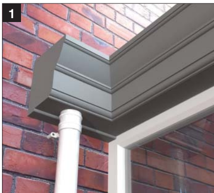
Return back to house wall applies to both Cornice and cill
